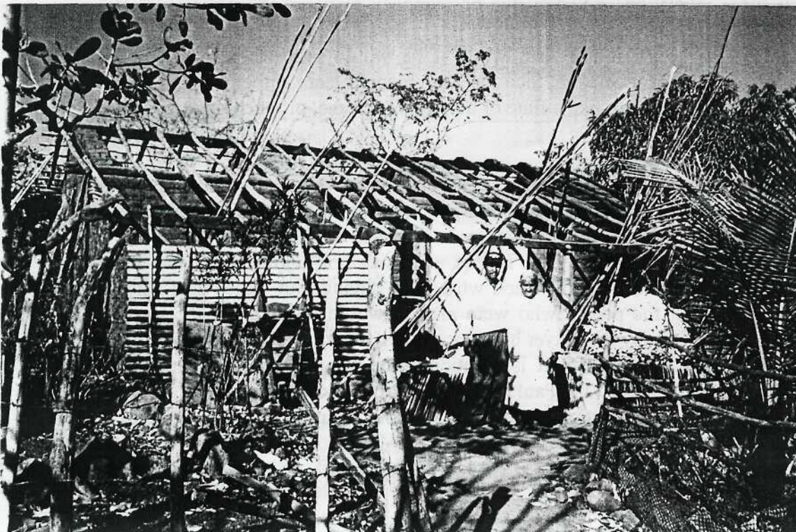
House of Brother Rivas was destroyed in the earthquake at Tequira, Usulután.
