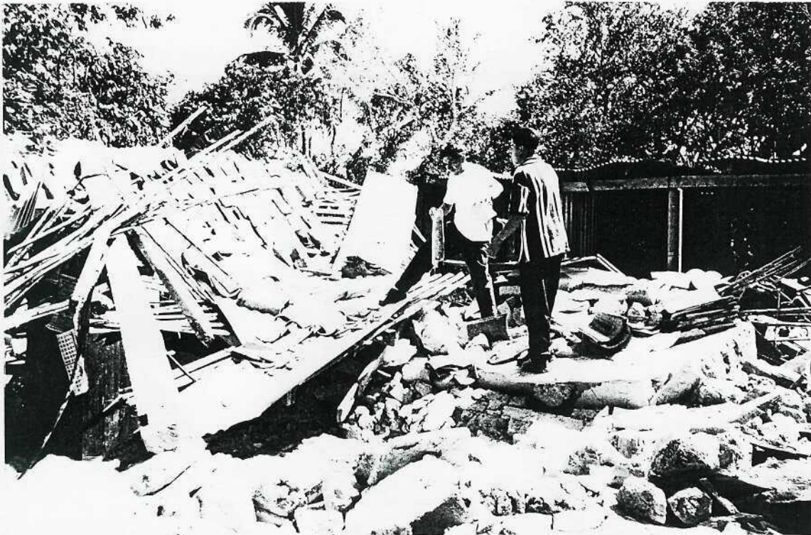
House of Brother Jose Carpio at Miraflores was destroyed
