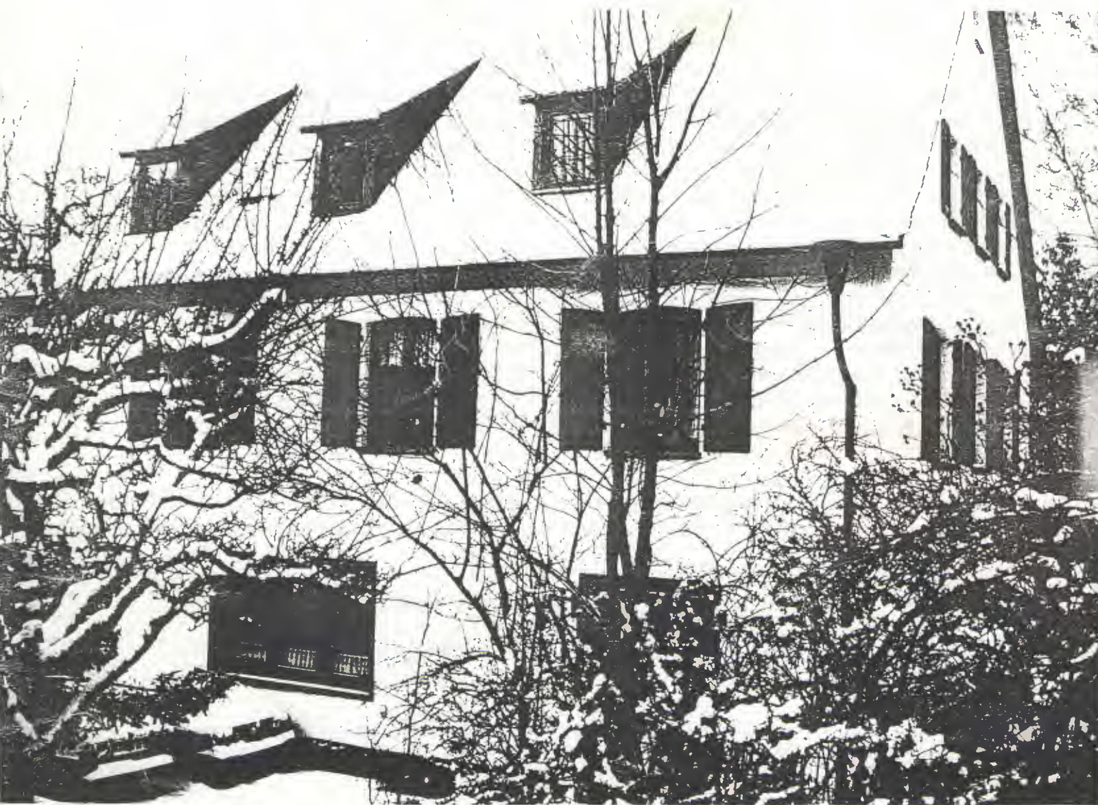
The General Conference Building at Mosbach, Germany.
